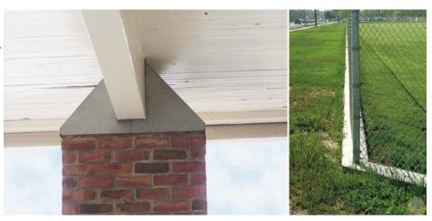
Less-toxic practices to prevent school pests include: *left*, designing buildings to prevent roosting pigeons, which can carry diseases, and, *right*, installing mowing strips to prevent weed growth along fence lines.
